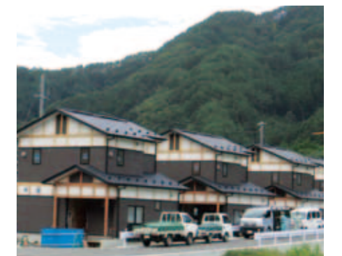
Public housing under construction (Otsuchi Town, September 2014)
