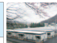
Temporary housing project (Kamaishi City)
