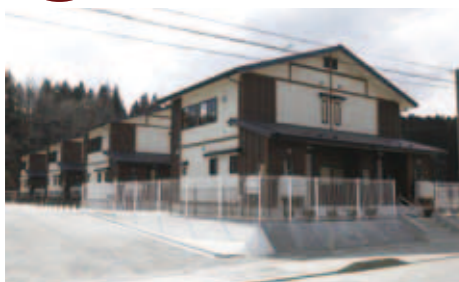
Public housing for survivors, building #1 in Monzen, Noda Village (completed on March 25, 2013)
