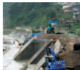
Kuji fishing port restoration work (Kuji City - September 2013)
