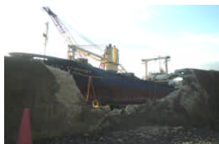
Top Photo : Asia Symphony swept to the pier dock. Left Photo : Damaged pier wall
