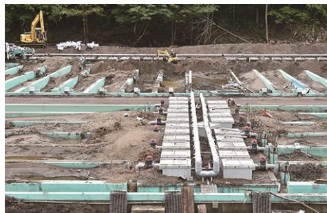
A salmon hatchery that was flooded and damaged (Noda)
