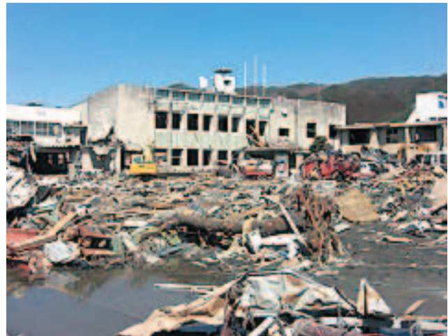
Otsuchi Town Hall was destroyed by the tsunami
