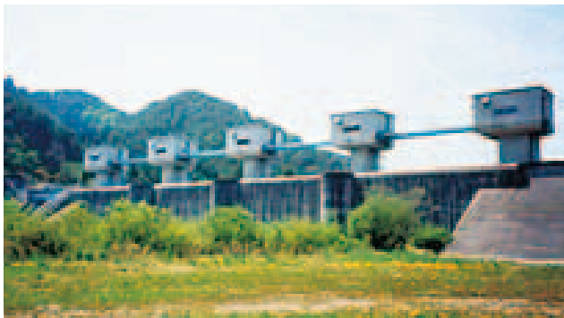
Floodgates that helped to mitigate damage from the tsunami in Fudai
