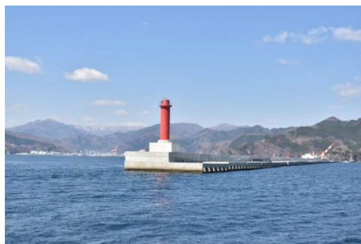
釜石港湾口防波堤
