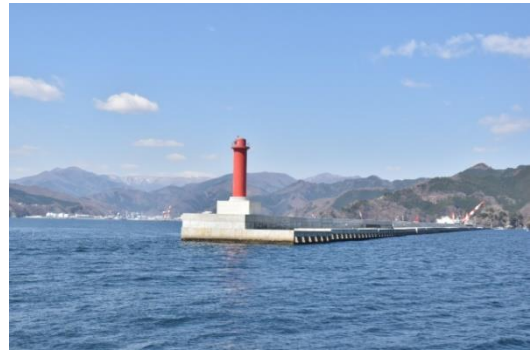
釜石港湾口防波堤
