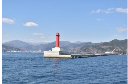
釜石港湾口防波堤
