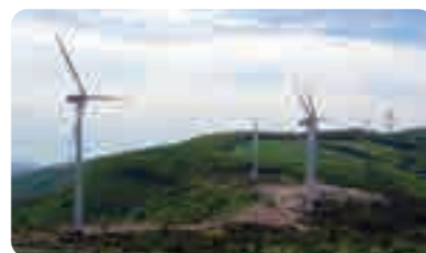
Wind power generation
