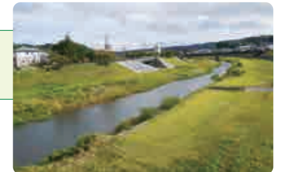
Construction was finished in 2004. The river became wider, and the riverbanks were made stronger
