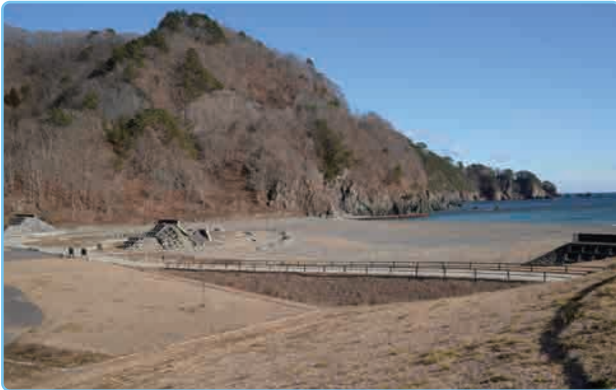
The broken seawall remains to show the terror of tsunamis
